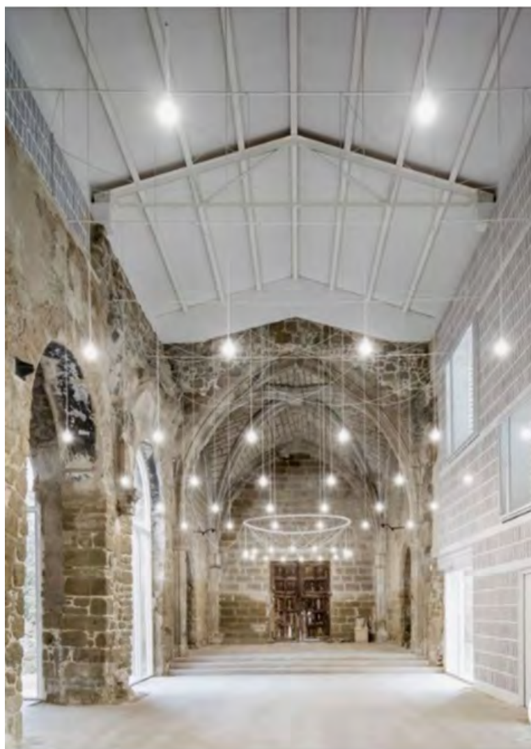
Figura 106: Sugestie vizuală: Santa María de Vilanova de la Barca / AleaOlea architecture & landscape. Photograph by Adrià Gouli
